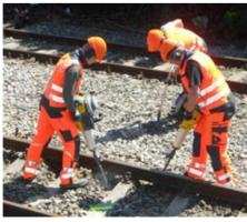
**Gasoline breakers BH40 and BH55rw** are specially optimized for maintenance work in railway construction.
